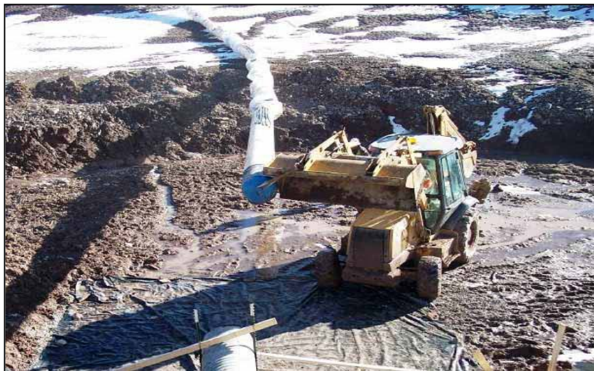
Figure B-24. —Guiding the 20-inch pipe into the upstream end of the CMP.
