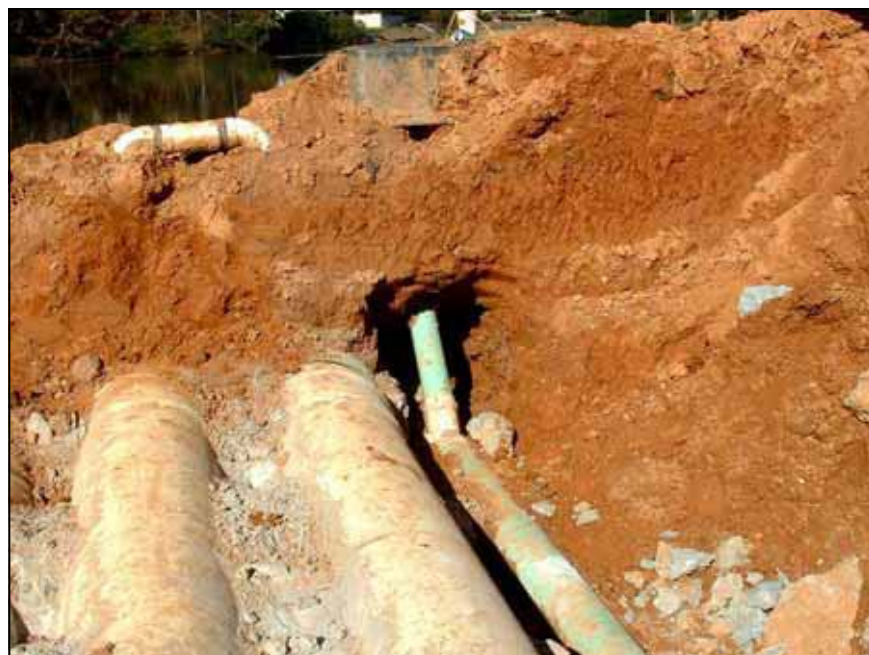
Figure B-13. —After about 10 years of operation, seepage was observed on the downstream slope of the dam in the vicinity of the siphons, and the overlying embankment material was excavated to expose the pipes to determine the source of the seepage.
