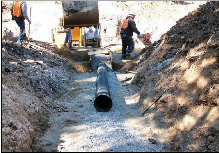
Figure 67. —Trapezoidal side slopes used in drainpipe construction.
