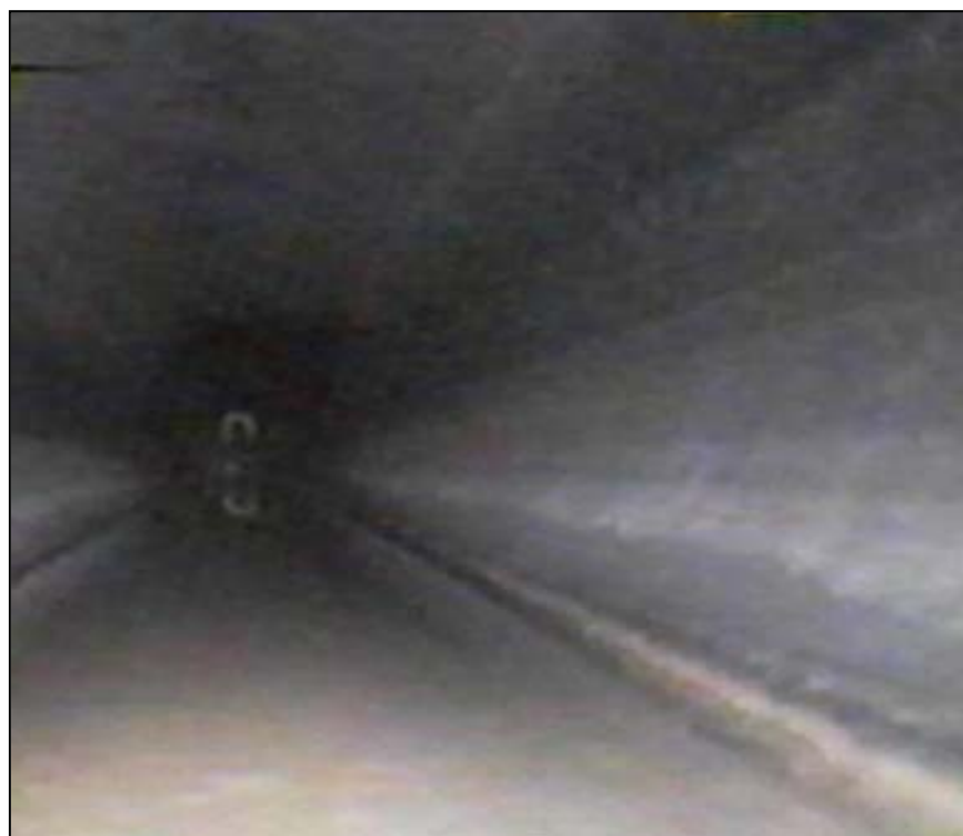
Figure 87. —Looking upstream toward the control gate in an HDPE sliplined outlet works conduit using CCTV inspection equipment.
