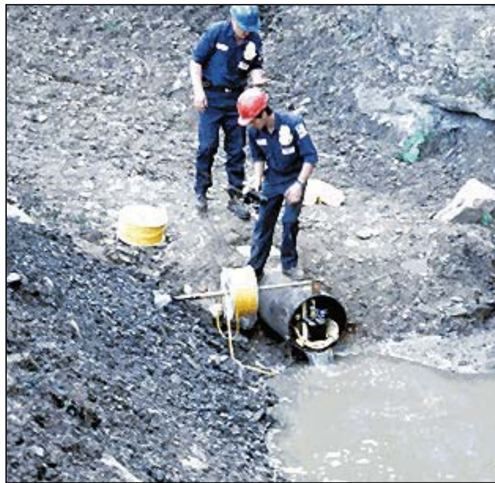
Figure 102. —Deflection monitoring of a decant pipe.
