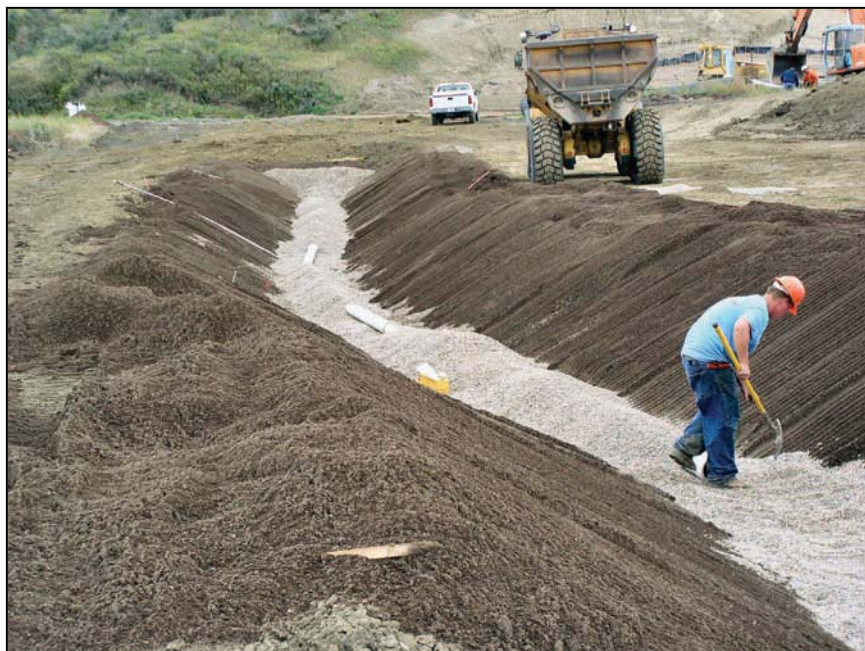
Figure 78. —Drain material being placed over a drainpipe.
