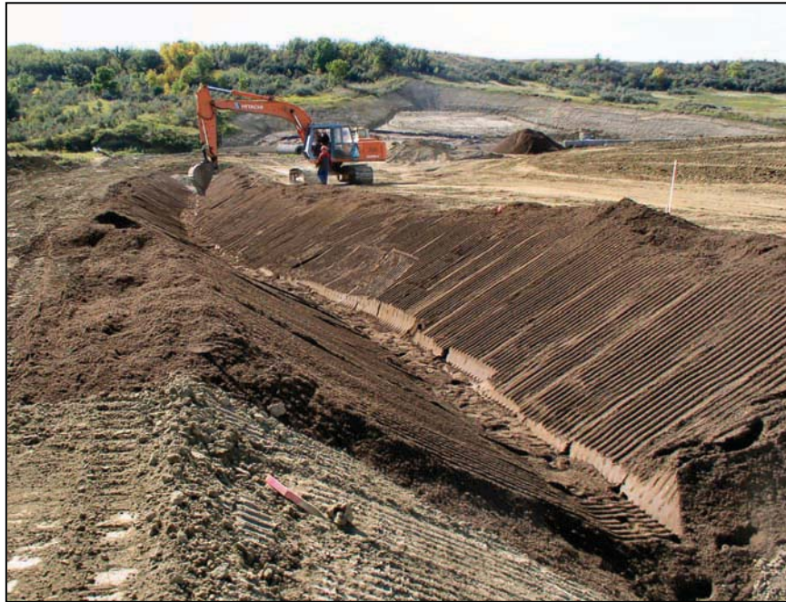
Figure 77. —Initial filter placement in a trapezoidal trench.
