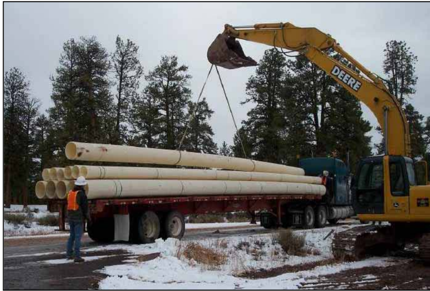
Figure B-23. —HDPE pipe being unloaded at the site using a John Deere 230LC excavator.
