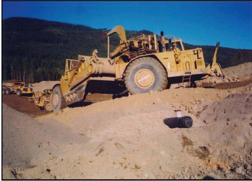
Figure 65. —Construction equipment can travel safely over plastic pipe when adequate cover above the drainpipe is provided.
