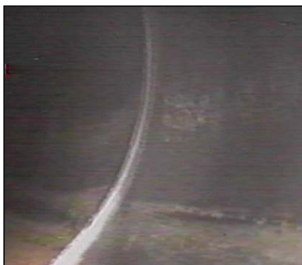
Figure 86. —A butt fused, solid walled HDPE pipe joint in an outlet works slipliner as viewed using CCTV inspection equipment.
