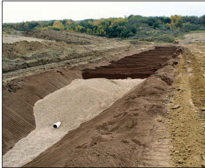
Figure 79. —Filter material being placed over drain material.
