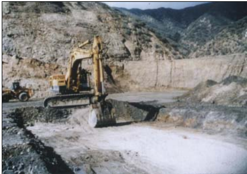
Figure 85. —Contaminated materials being excavated beneath a roadway crossing over a filter. Photo courtesy of ASDSO (Hammer, 2003).
