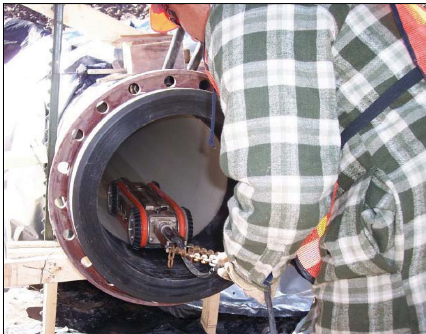
Figure 88. —CCTV inspection of a newly installed slipliner for an outlet works renovation.
