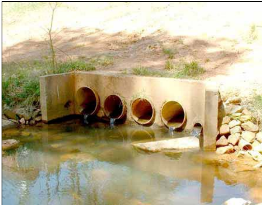
Figure B-12. —In the early 1990's the spillway capacity of the dam was increased by construction of a system of 5 PVC siphons embedded in concrete in a shallow trench through the dam.
