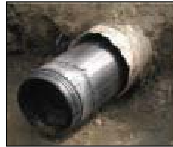
Figure 13. —Male end of snap joint.
