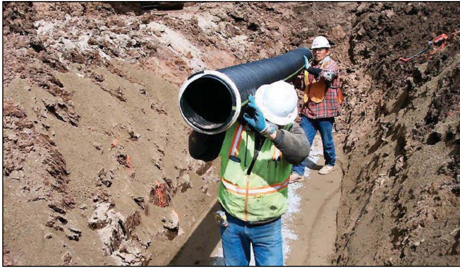
Figure 1.—Plastic pipe is lightweight, which facilitates installation.
