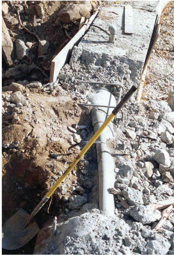
Figure B-17. —Looking downstream from toe of dam after excavation of collapsed portion of HDPE pipe (located in original box conduit, upstream of new concrete encasement).
