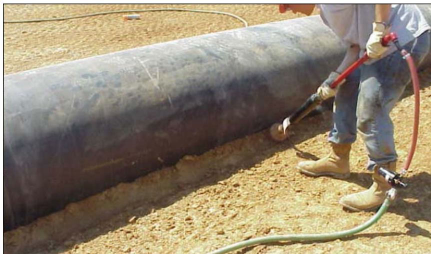
Figure 49. —Compacting earthfill under the haunches of plastic pipe is very difficult and quality compaction can not be achieved.
