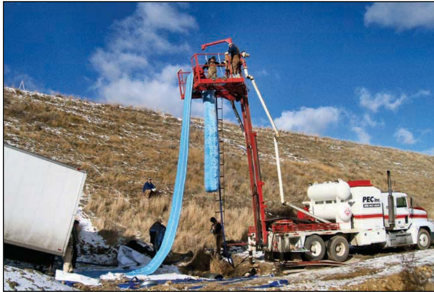
Figure 22. —Contractor installing a resin-soaked CIPP liner into an existing outlet works. Installation begins by hauling the liner up to the top of the platform. On the platform, water is run into the liner causing it to pressurize and expand downward. As the liner reaches the outlet works pipe opening, laborers on the ground maneuver the water filled liner into the outlet works. Water pressure continues to cause the liner to advance upstream in the outlet works pipe and un-invert itself. Photo courtesy of Tetra Tech Inc.
