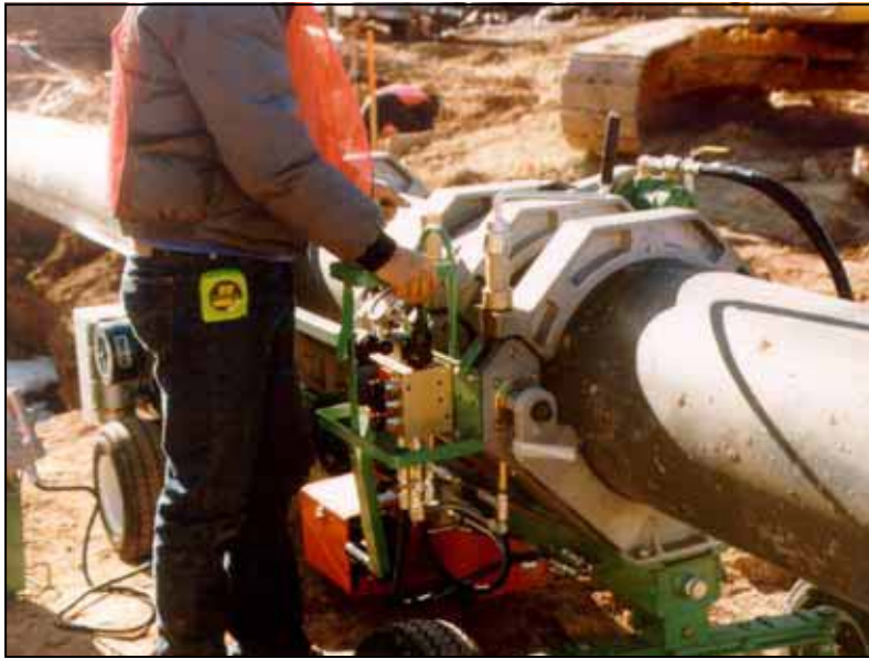
Figure 9. —HDPE pipe joint being butt fusion welded.
