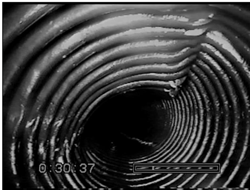
Figure B-3. —A buckled left toe drain pipe at approximately Sta. 23+25 stopped the camera-crawler. A cleaning removed fine materials from the pipe invert.
