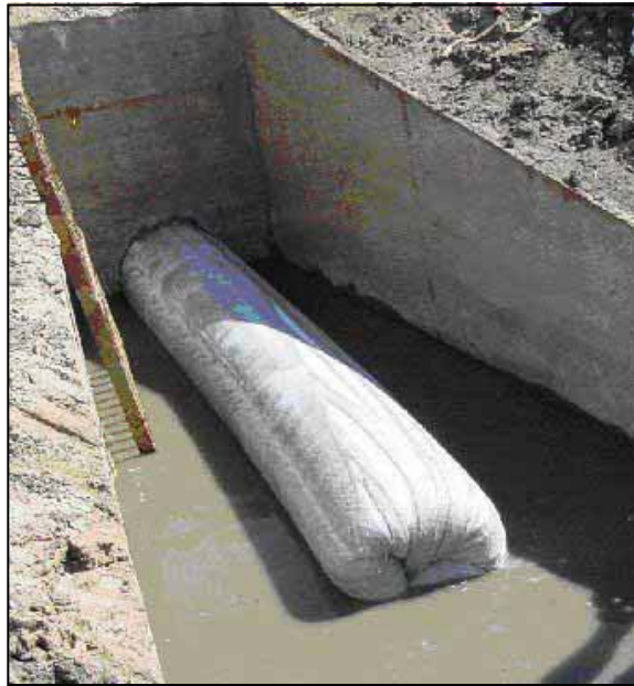
Figure 21. —CIPP liner exiting from an existing outlet works conduit, via the hydrostatic inversion method.
