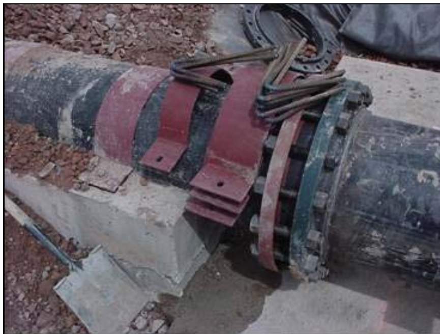
Figure 50. — Until further research is completed, concrete cradles beneath plastic pipe should not be used.
