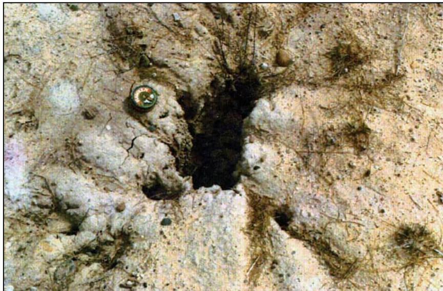
Figure B-4. —Subsurface fissure located at the downstream toe of the dam east of the outlet works. The subsurface soil had a very high moisture content.
