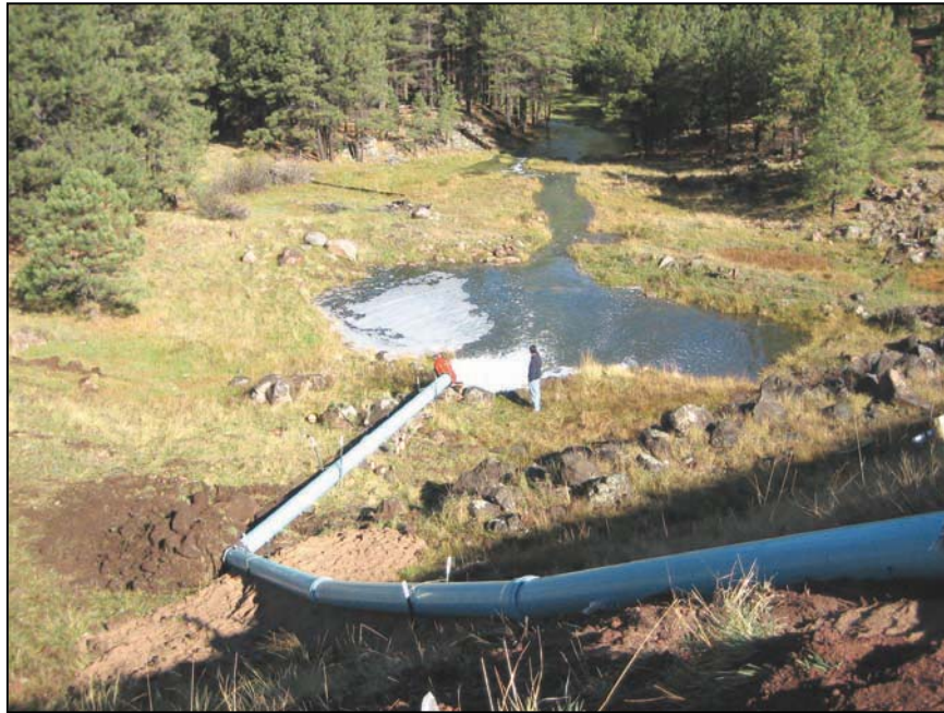
Figure 25. —A temporary siphon constructed using PVC pipe. This siphon is being used for short term operation.
