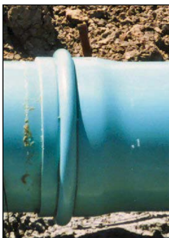
Figure 16. —PVC pipe joint (bell and spigot).
