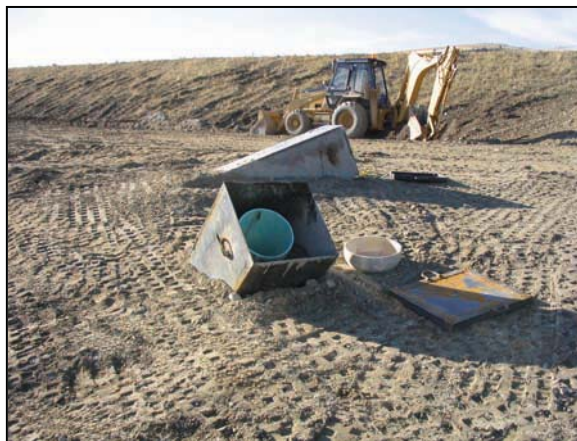
Figure 61. —A drainpipe cleanout with a steel encasement and lockable protective cover.
