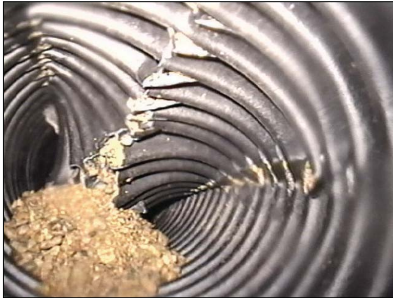
Figure 45. —Single wall corrugated HDPE drainpipe experiencing failure due to buckling.
